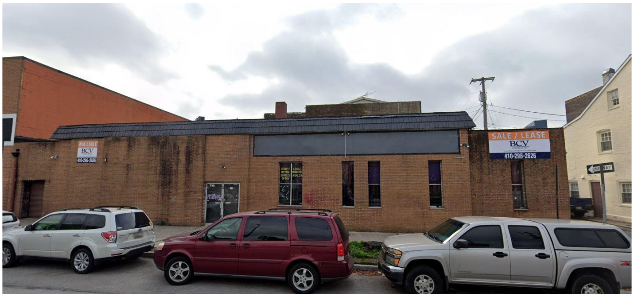
Exhibit 10. Google streetview Eastern Avenue, 2020
